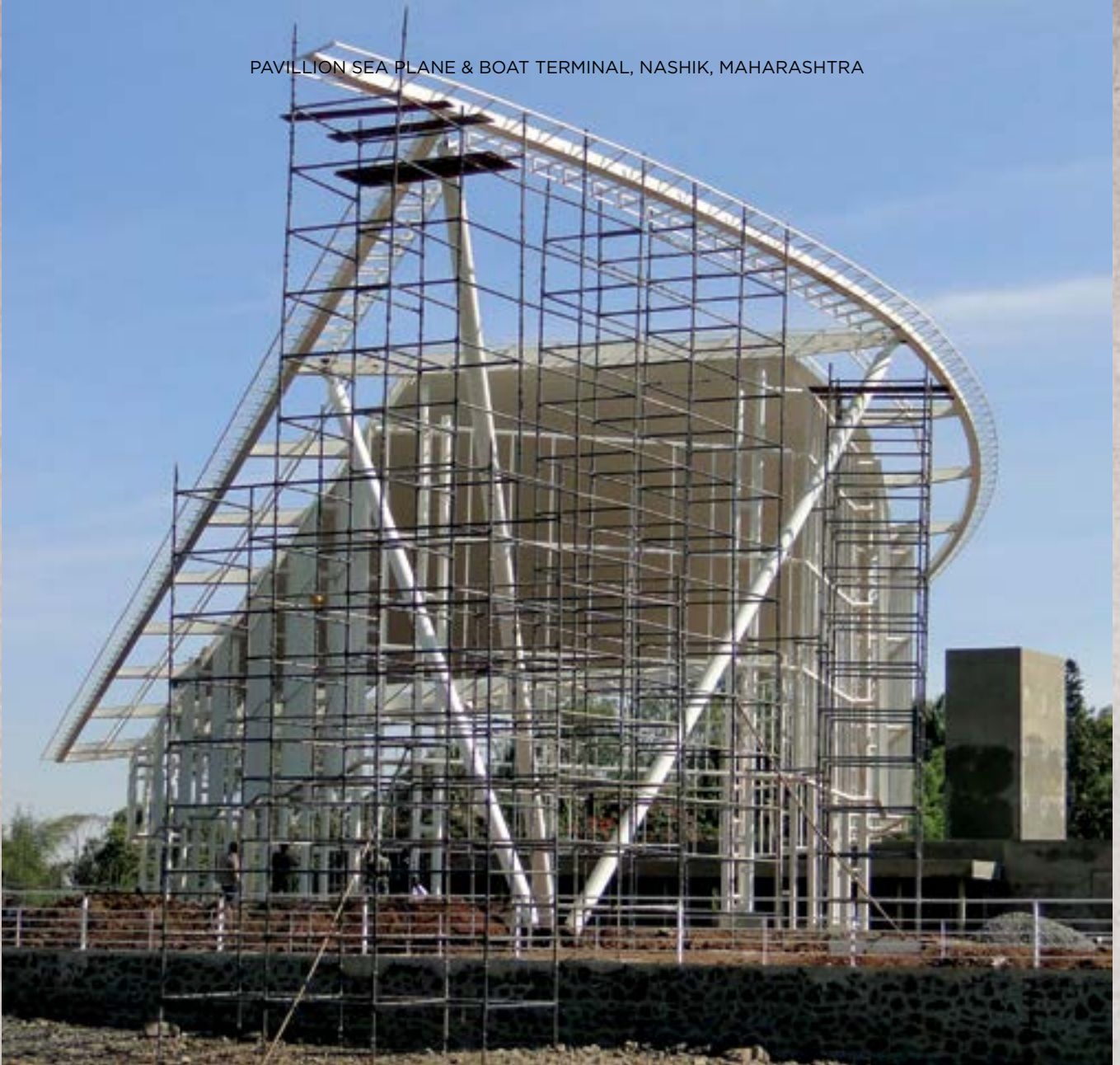
Fig #6: Anchor columns under installation
