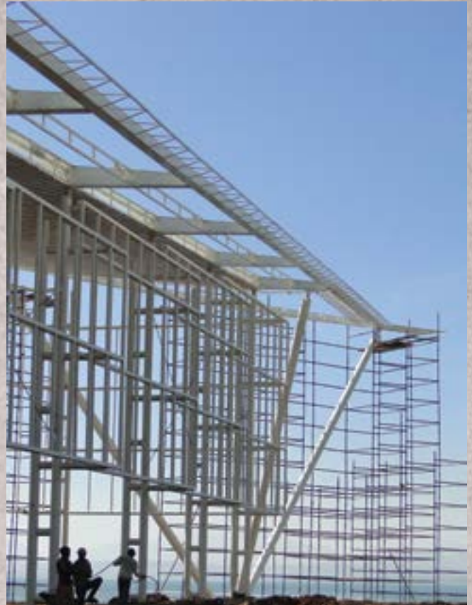
Fig #11: Dual Steel Columns under construction1
