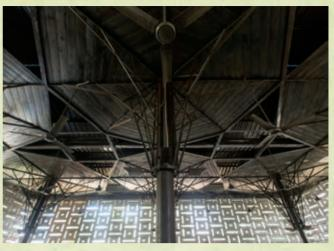
Fig #13: Tree branch column holding the umbrella shapped ceiling
