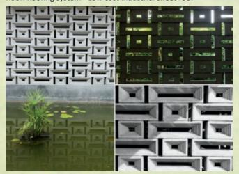
Fig #10: Custom-made perforated CC block wall
