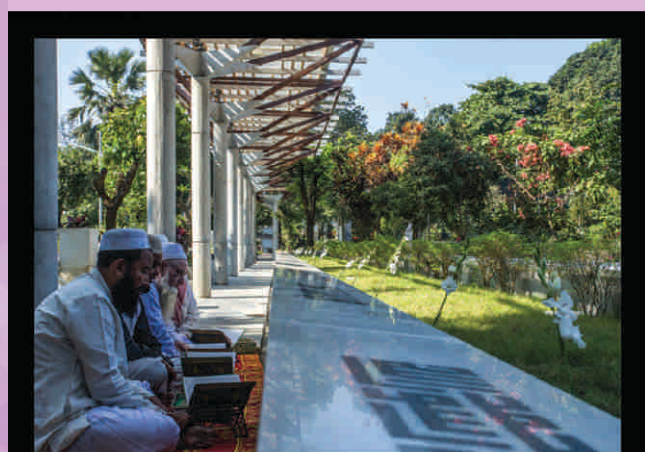
Shading created with light materials on the walkways in front of the graves for public access while keeping the transparency for light and air flow
