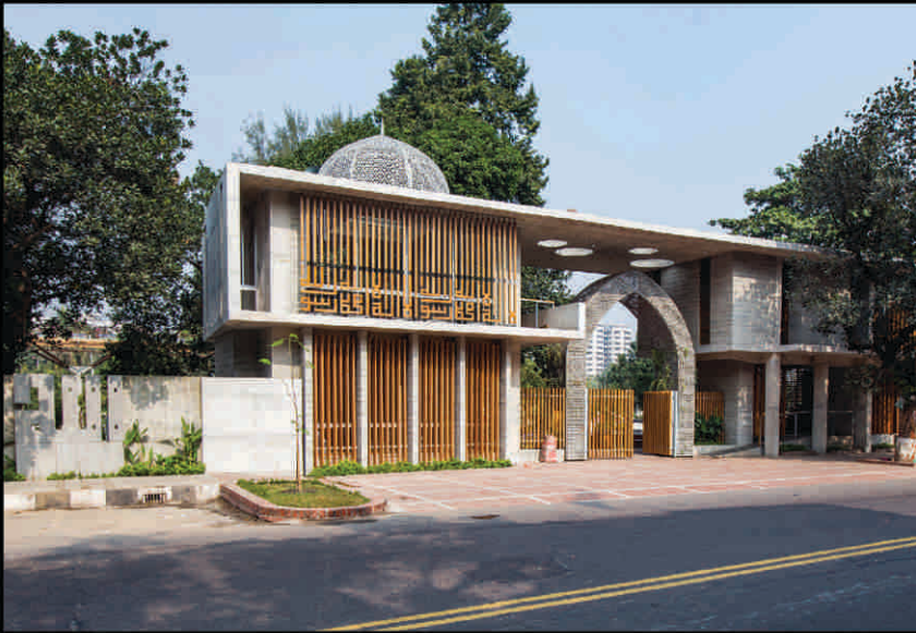
Wooden Louvers and metal screens delimited gatehouse as a representation of the traditional patterns
