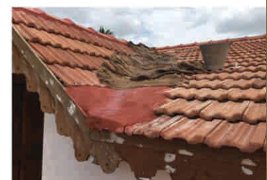
Valley - Terracota tiling over main roof
