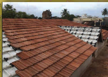
Terracota Tiling in process over main roof
