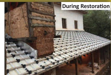
Laying of TRIMDEX over wooden boardings
