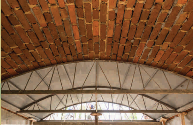
Figure 8: Segmental vaulted roofing in bricks
